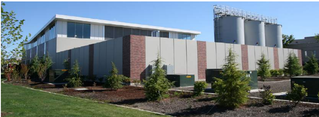
Left: Energy Center
