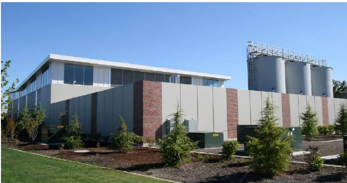
First LEED Platinum Energy Plant
